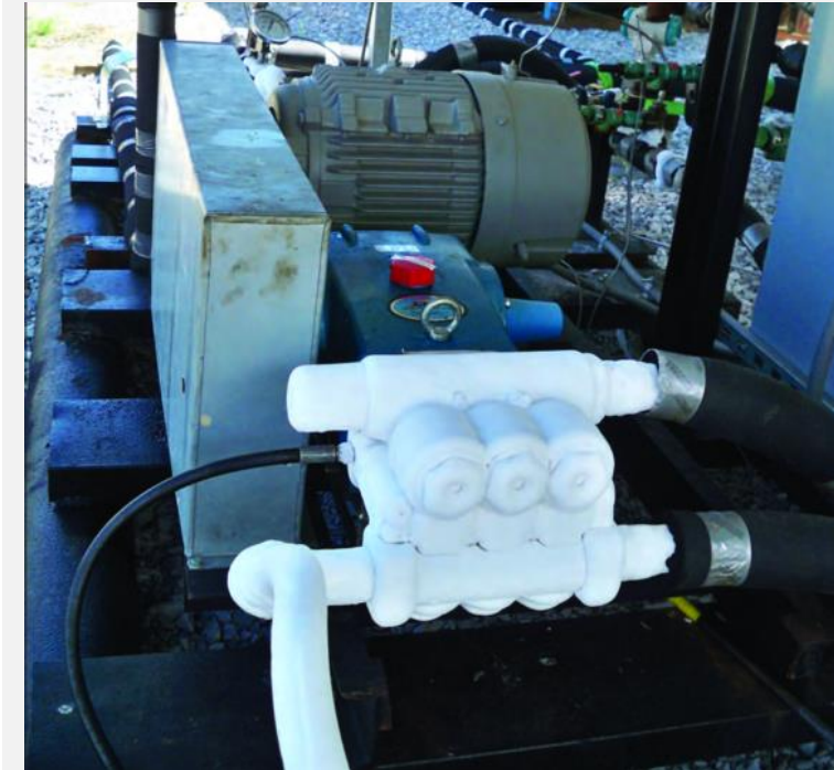
Typical Triplex C02 Injection Pump
