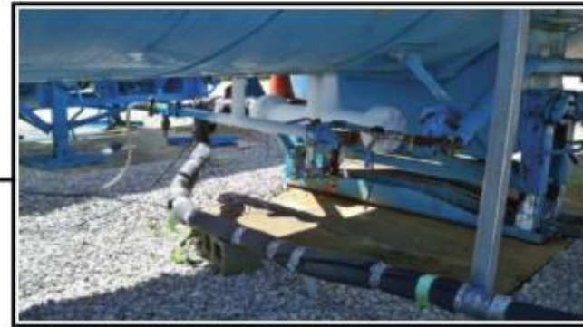
Figure 2 CO2 storage tank connections at site. Frosted-over 4-inch tee going to black hose is liquid CO2 supply. The black hose is an insulated line to the booster pump suction
