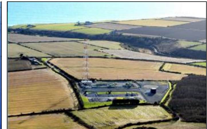
Onshore gas terminal and Entry Point to Gas Networks Ireland gas grid. Terminal tariff based on operating costs for gas throughput
